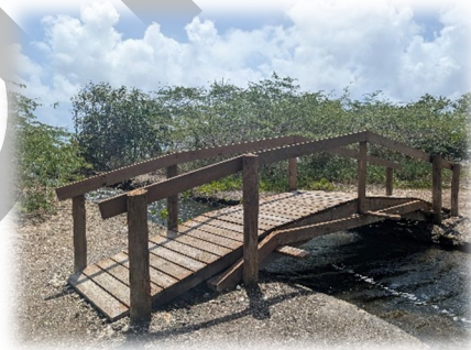
Figure 16. Wooden Bridge Across a Hydrological Connection Channel
